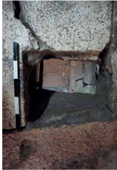
Fig. 4b. View of the manhole after excavation.
